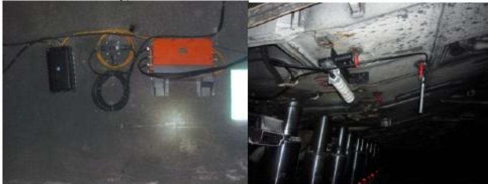
Figure 6. Base station installation on site
